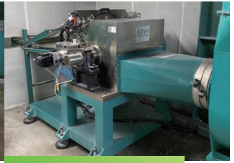
Direct release to storage tanks after shredding
