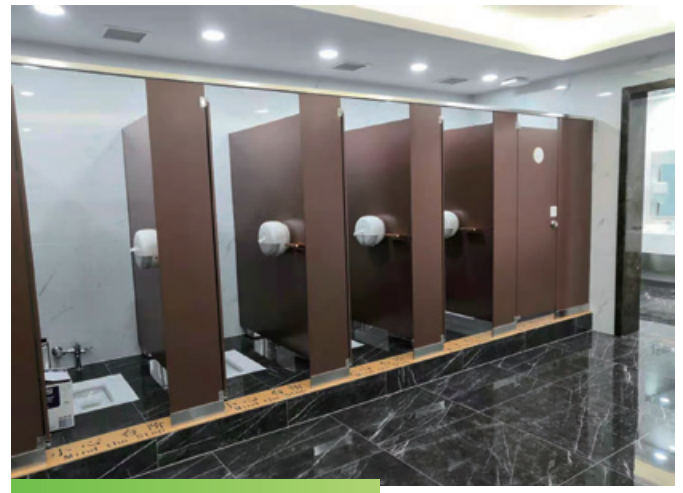
Public restrooms fulfilled by Tork at Shijiazhuang Zhengding International Airport
